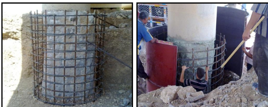
Figure (5) Placing of Steel Mesh and Steel Casing (Before Concrete Poured)
