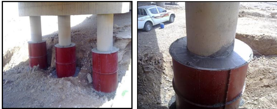
Figure (7) Treatment of damaged joints by RC Confined by Steel Casing (After Concrete Poured)
