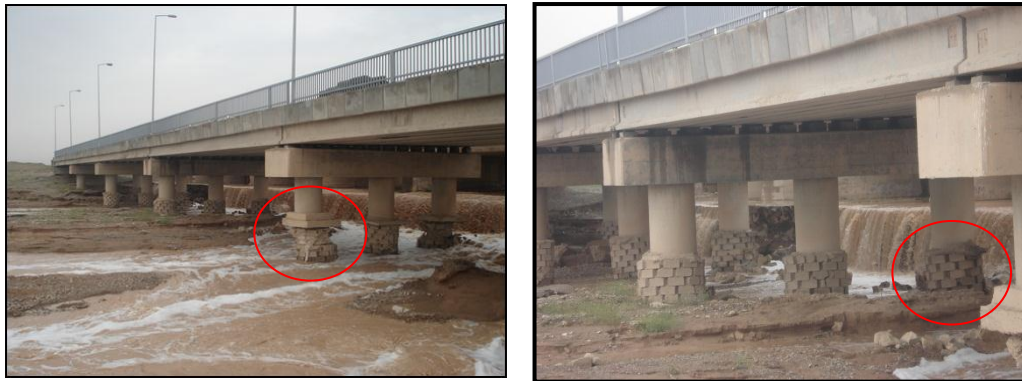
Figure (1) Damages at the Heads of Piles (Joint) and at Aspects
