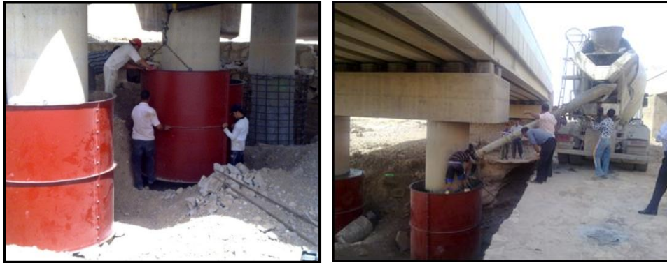
Figure (6) Steel Casing (Molds) and Concrete Poured (Concrete Pumping)
