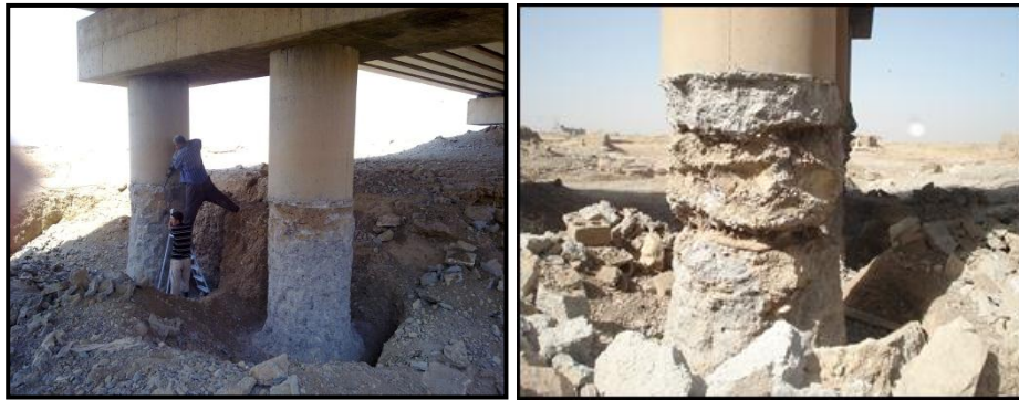
Figure (4) Preparation of Joints (Removing of weak Layers)
